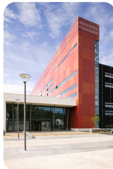
The snus manufacturing facility in Kungälv, Sweden, opened in 2003 and was expanded in 2009 and 2010.
