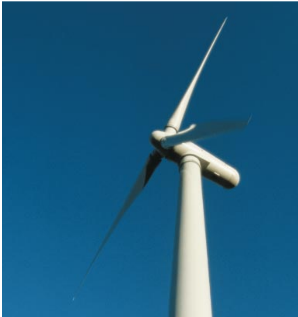
The wind power plant, Elin, supplies nearly 20 percent of the energy needs for Swedish Match's snuff plant in Gothenburg.
