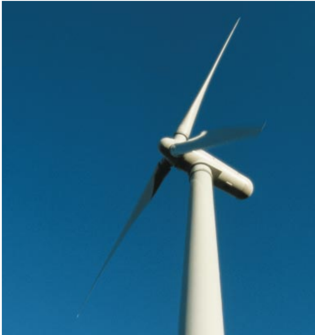
The wind power plant, Elin, supplies nearly 20 percent of the energy needs for Swedish Match's snuff plant in Gothenburg.
